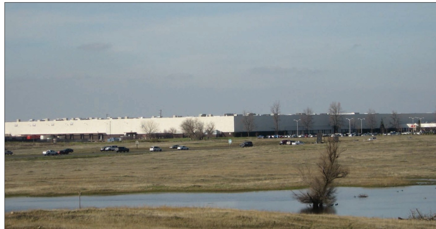
PHOTO 4 ACE Hardware Warehouse Facility (facing northwest).
