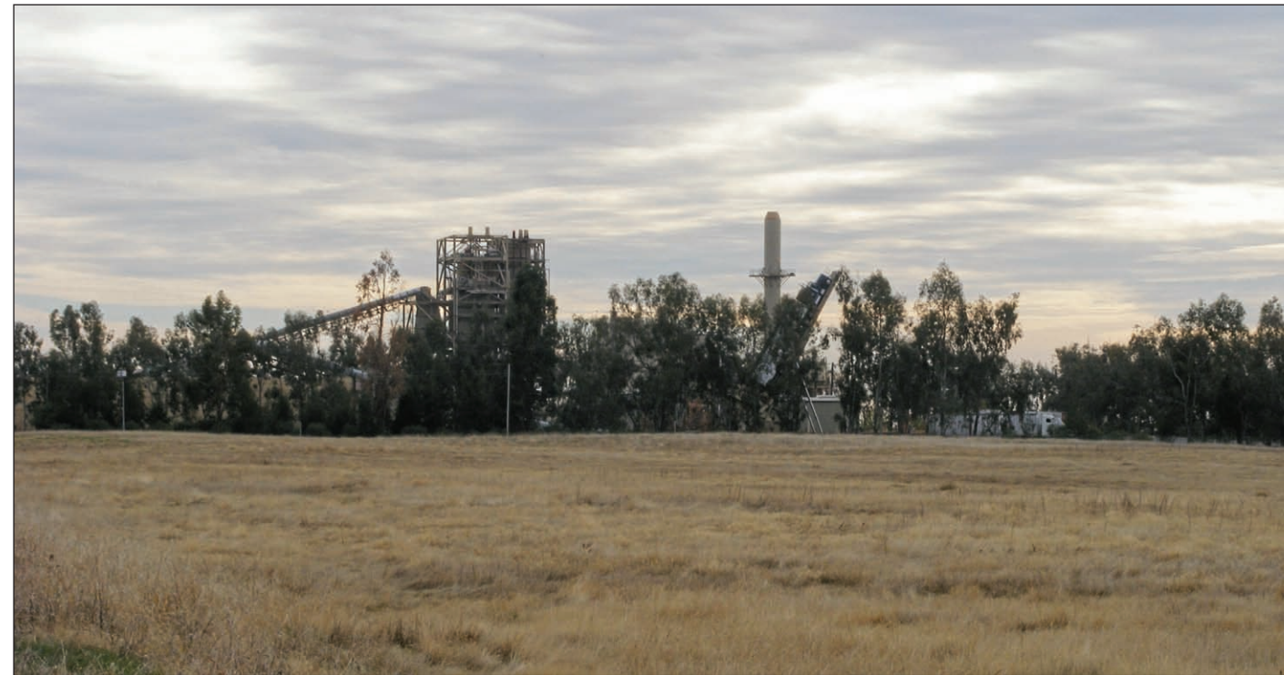
PHOTO 2 Rio Bravo Rocklin Biomass Power Plant (facing south).
