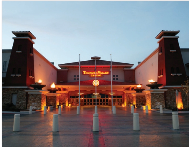
Thunder Valley Casino is an approximately 237,000 square foot facility that includes video gaming and card tables, four restaurants, five fast food outlets, and two lounges.
